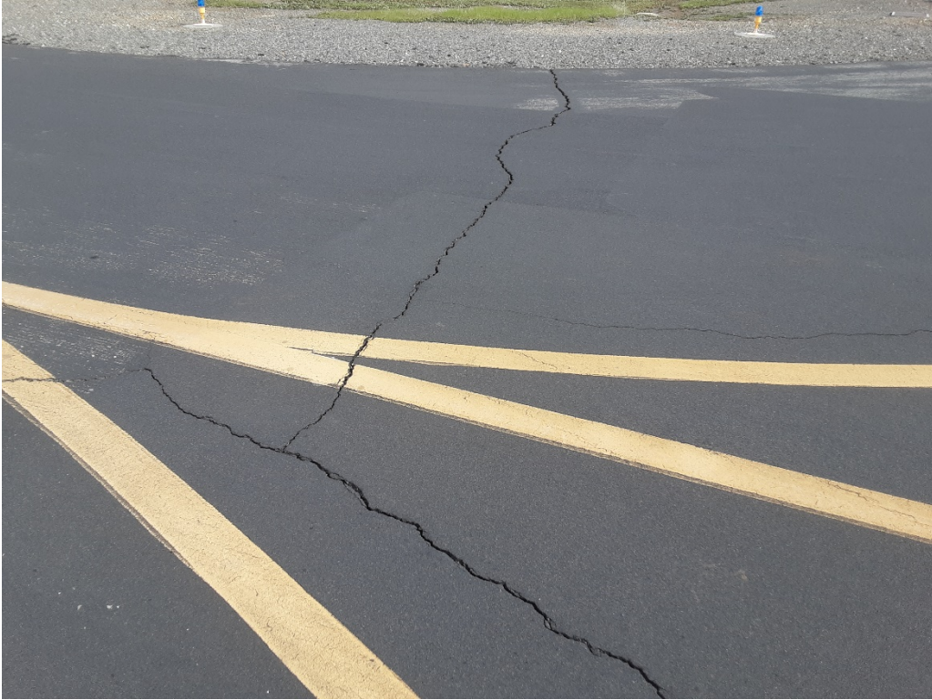
T8 B. LT cracking (Sample Unit No. 01).
