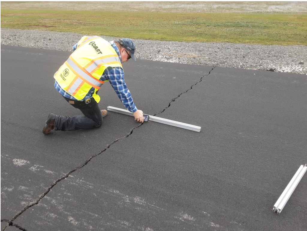
R1 B. LT cracking (Sample Unit No. 25).
