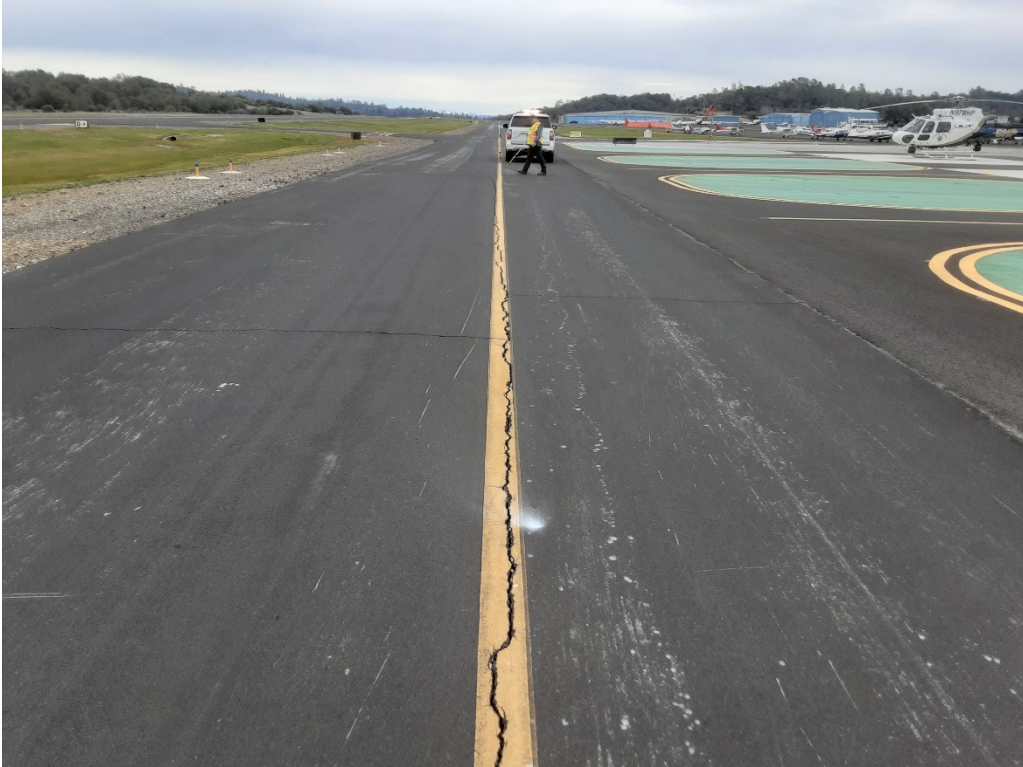
T1 A. LT cracking (Sample Unit No. 12).
