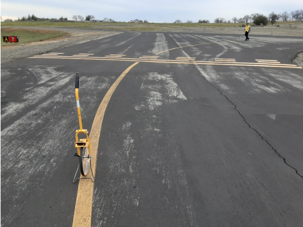
T3 A. LT cracking (Sample Unit No. 01).
