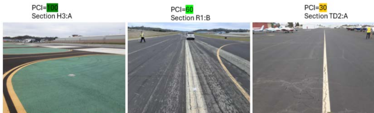
Figure 4. Example of PCI versus Pavement Condition
