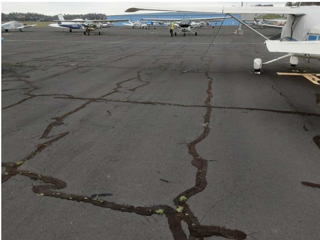
TD1 A. Block and LT cracking (Sample Unit No. 32).
