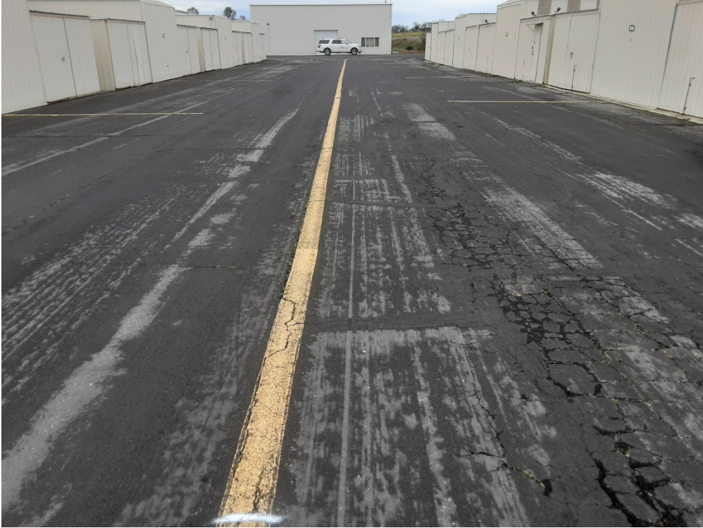
TD4 A. Alligator and LT cracking (Sample Unit No. 02).
