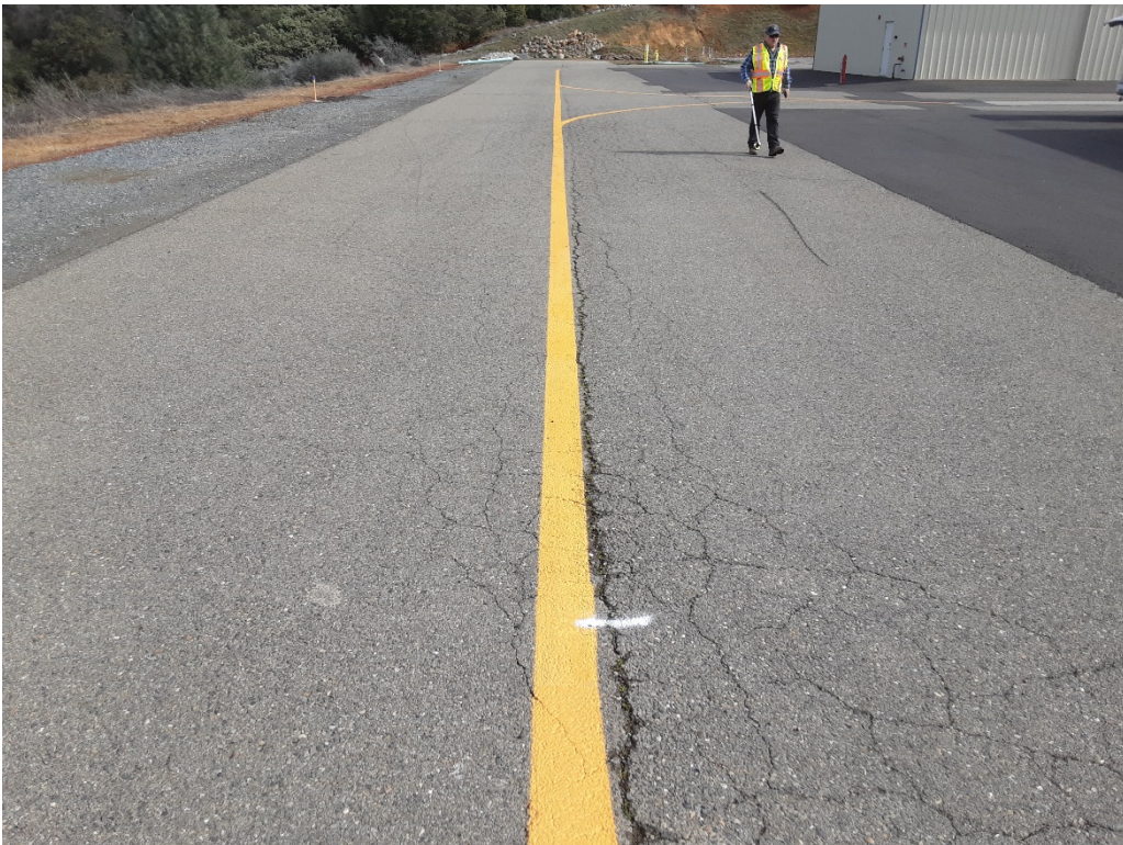
A8 A. Alligator and LT cracking (Sample Unite No. 19).
