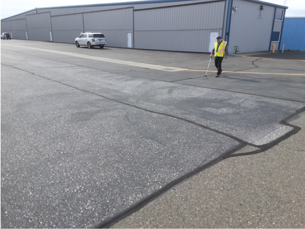
A8 A. LT cracking filled (Sample Unite No. 06).
