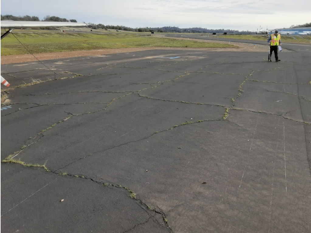
A3 A. Block and LT cracking (Sample Unit No. 02).
