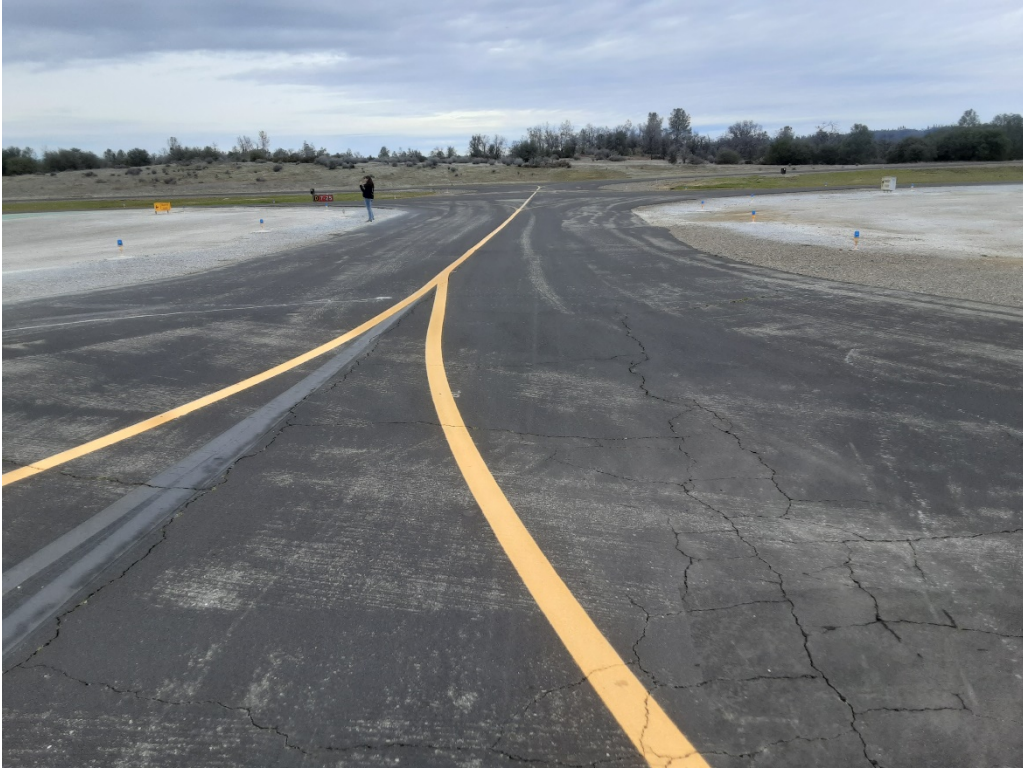
T2 B. LT cracking (Sample Unit No. 01).
