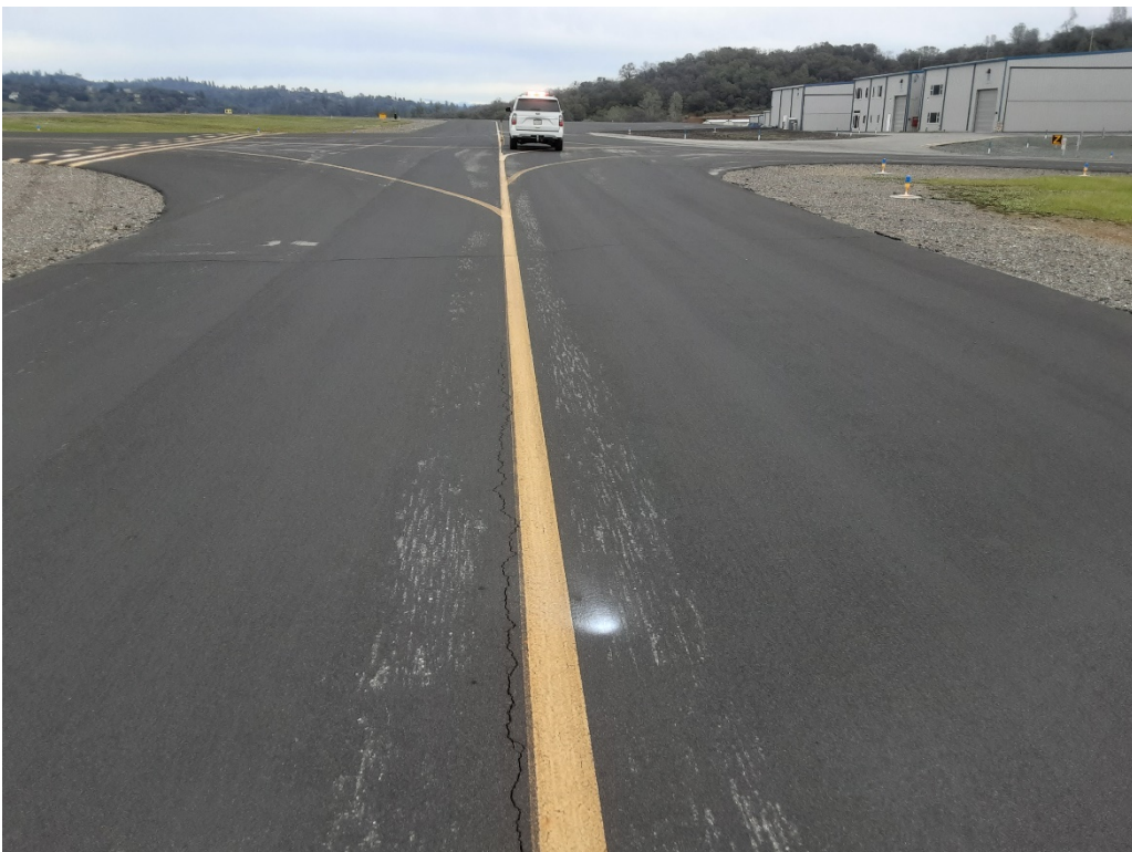
T1 A. LT cracking (Sample Unit No. 30).
