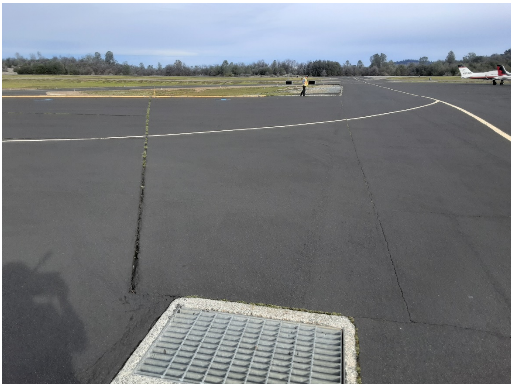
A1 B. LT cracking (Sample Unit No. 01)
