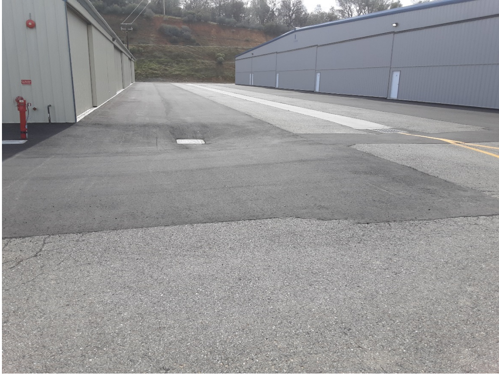
A8 A. Alligator cracking and patching (Sample Unite No. 19).
