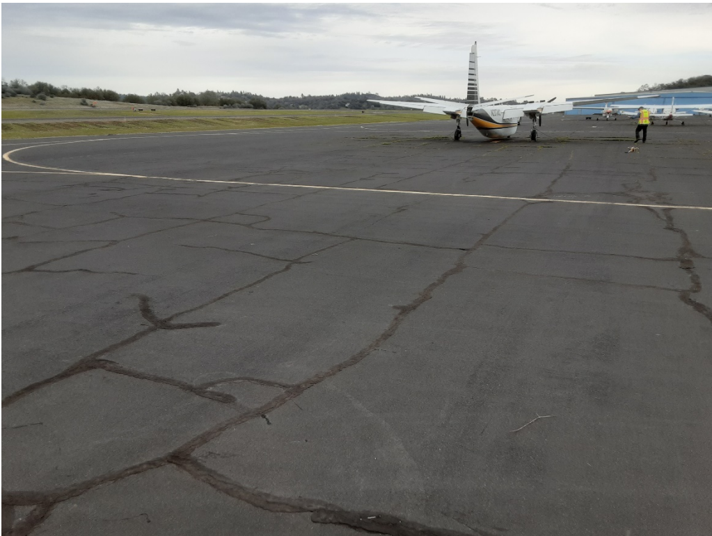
TD1 A. Block and LT cracking (Sample Unit No. 09).
