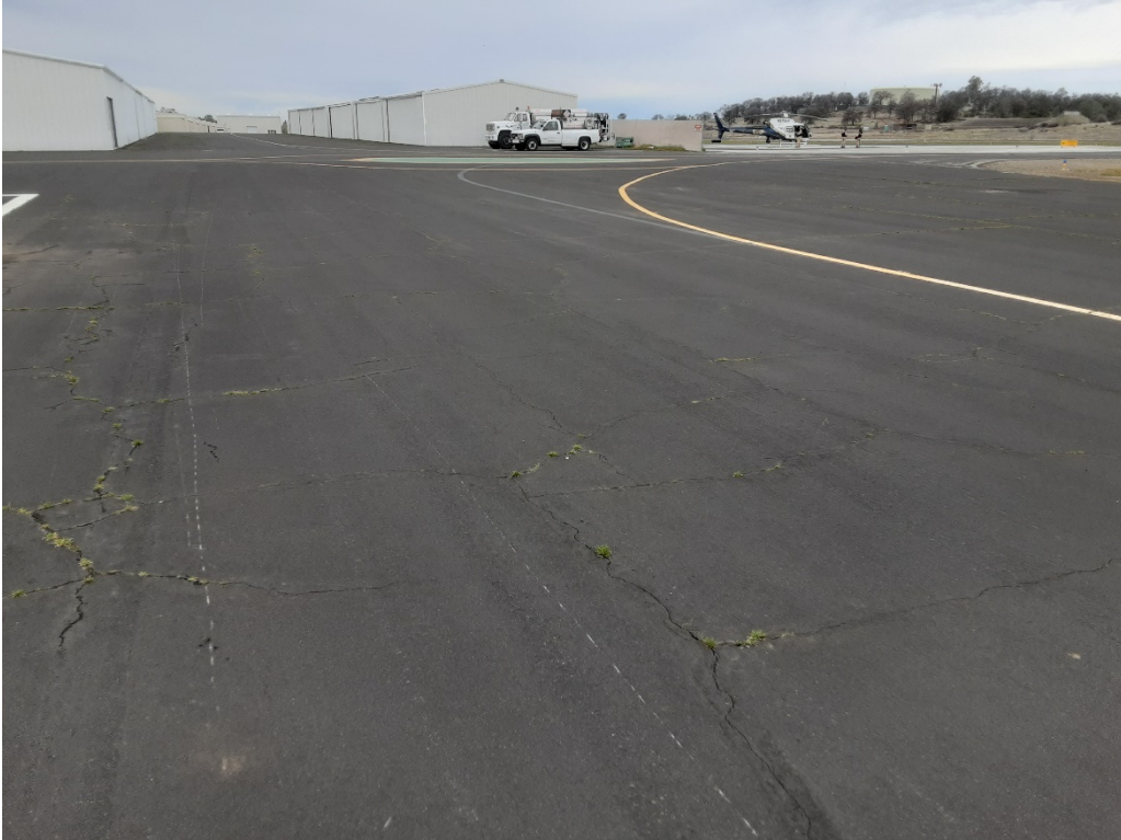
TD2 A. Block and LT cracking (Sample Unit No. 06).
