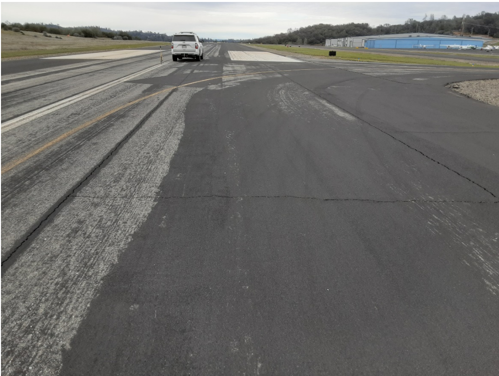
R1 B. LT cracking (Sample Unit No. 34).
