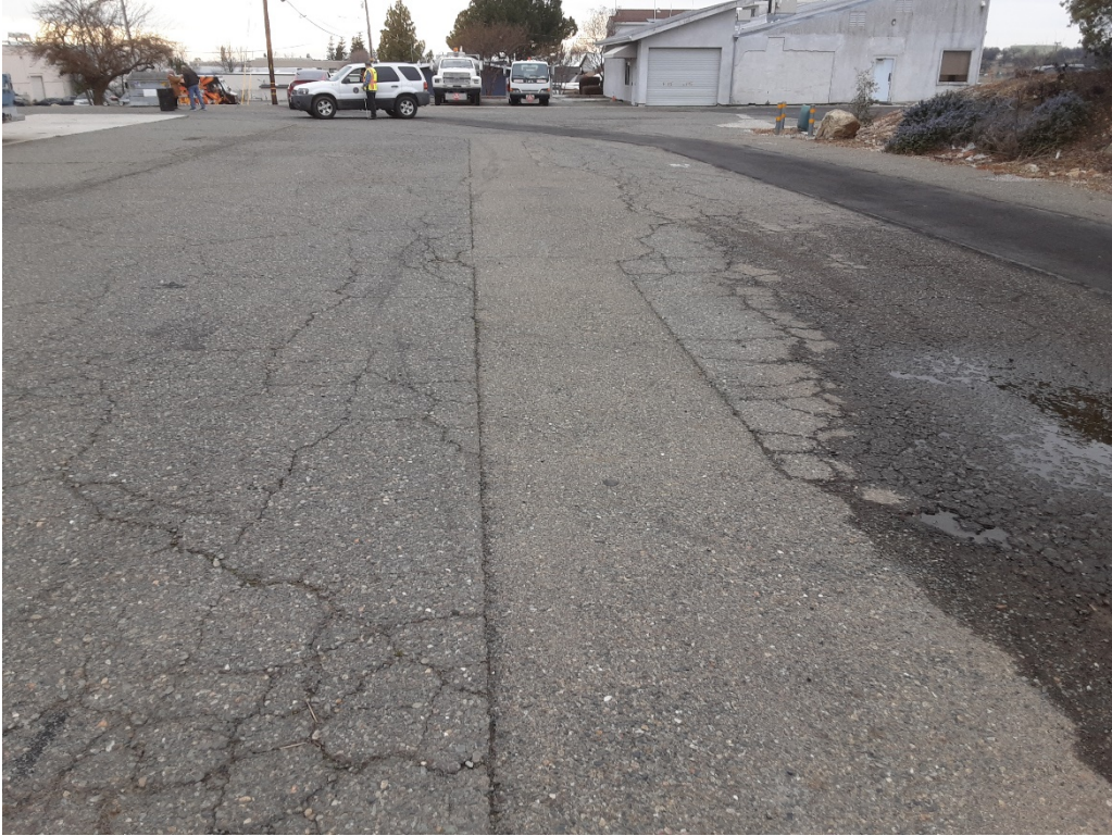
A9 A. Alligator cracking, patching and LT cracking (Sample Unit No. 02).
