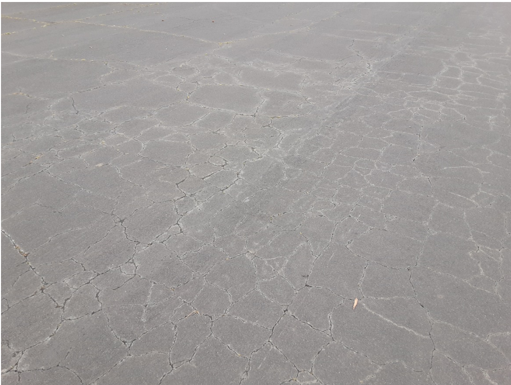
TD2 A. Alligator cracking (Sample Unit No. 17).
