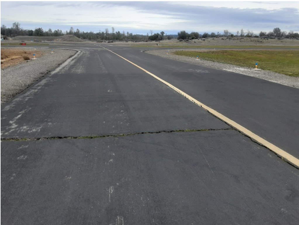
T6 B. LT cracking (Sample Unit No. 01).
