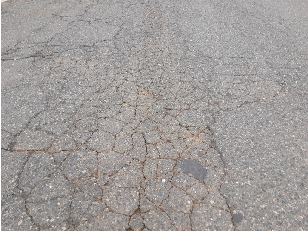
A9 A. Alligator cracking (Sample Unit No. 06).
