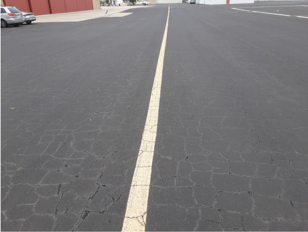
TD2 A. Alligator cracking (Sample Unit No. 17).
