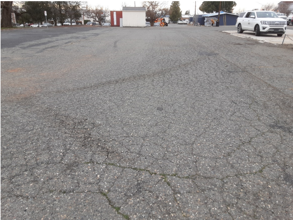
A9 A. Alligator cracking (Sample Unit No. 06).
