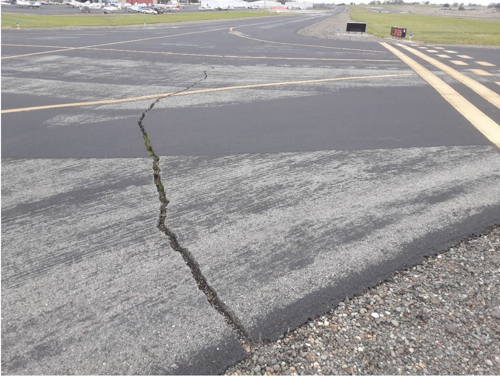
T8 A. LT cracking (Sample Unit No. 01).
