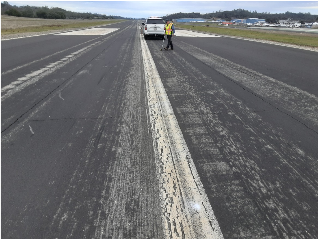
R1 B. LT cracking (Sample Unit No. 16).
