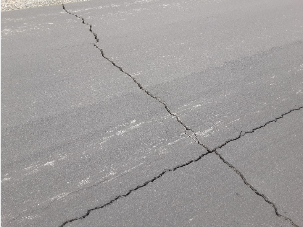
R1 B. LT cracking (Sample Unit No. 38).
