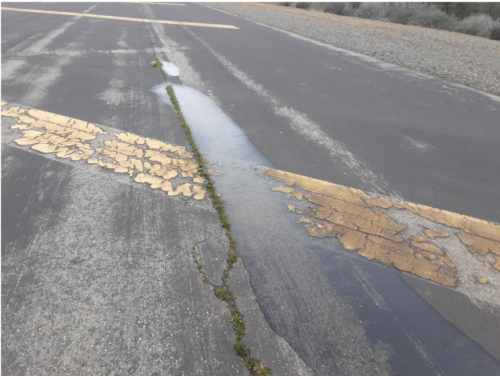
R1 C. LT cracking with moisture under the pavement (Sample Unit No. 03).
