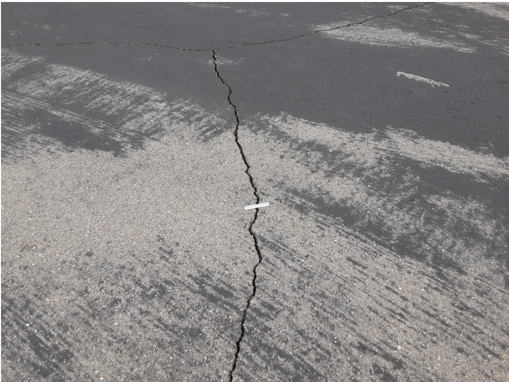
A5 A. LT cracking (Sample Unit No. 01).
