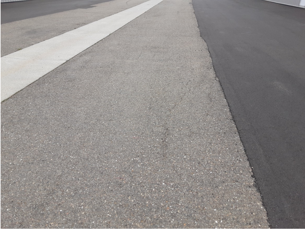
A8 A. LT cracking (Sample Unite No. 22).
