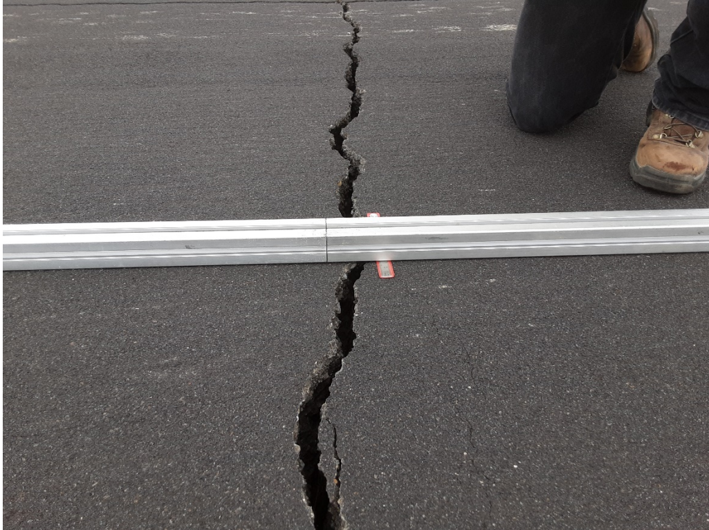
R1 B. LT cracking with faulting (Sample Unit No. 25).
