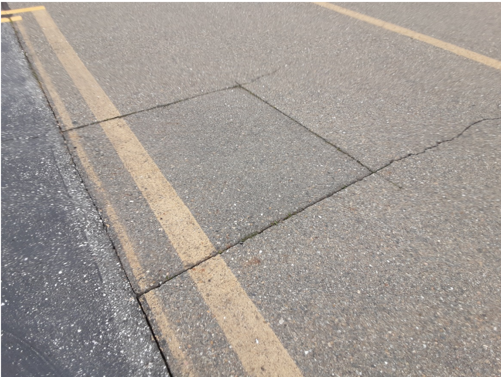
A8 A. LT cracking (Sample Unite No. 02).
