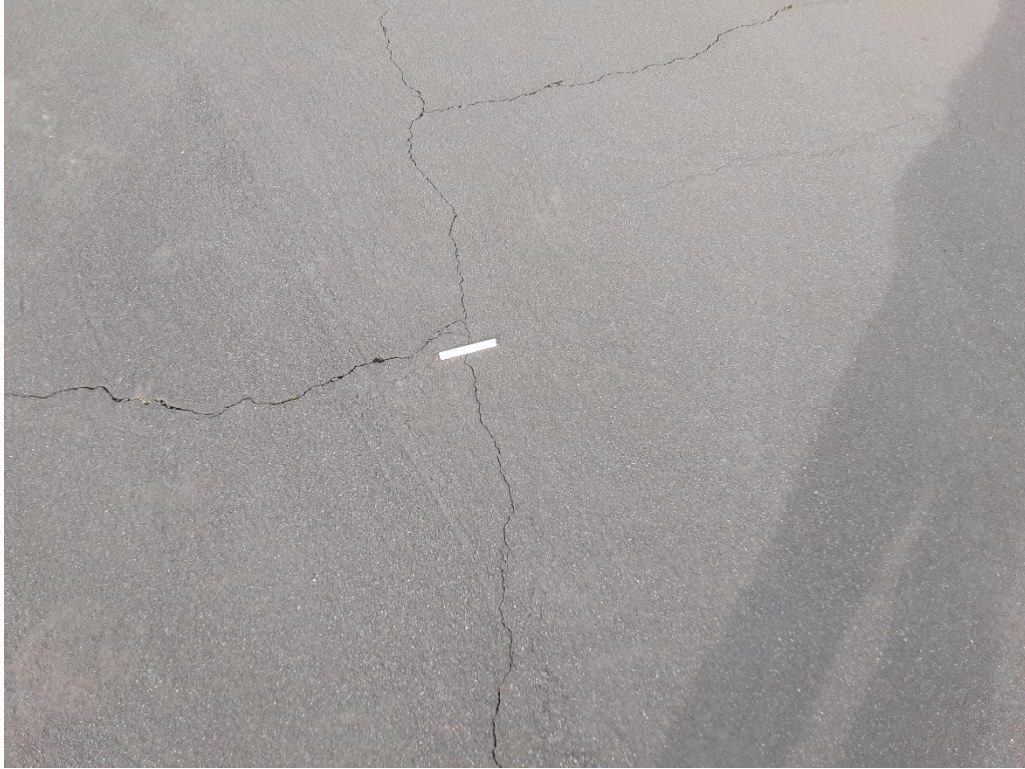
A1 B. LT cracking (Sample Unit No. 01)
