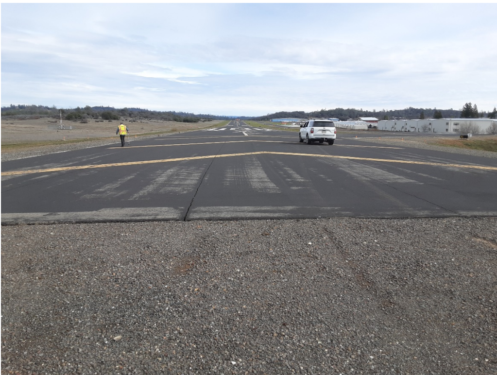
R1 A. LT cracking (Sample Unit No. 01).
