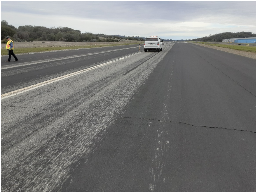
R1 B. LT cracking (Sample Unit No. 29).
