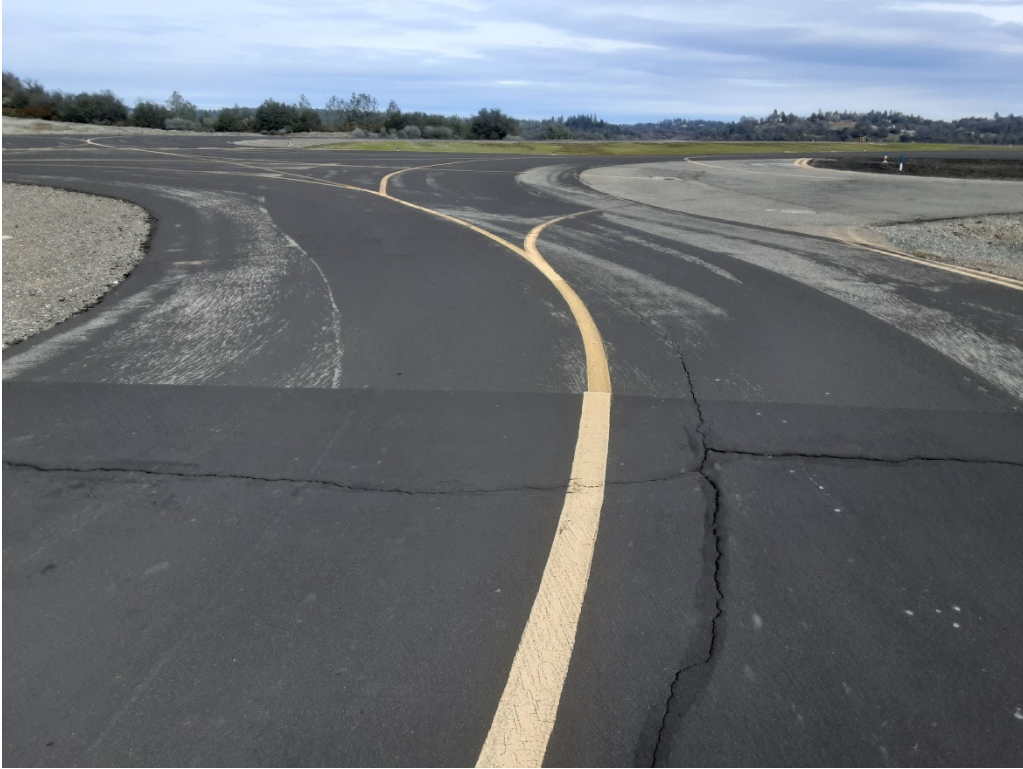
T4 B. LT cracking (Sample Unit No. 01).
