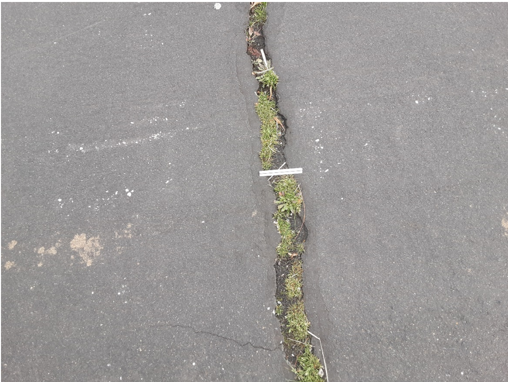
A1 A. LT cracking (Sample Unit No. 01)
