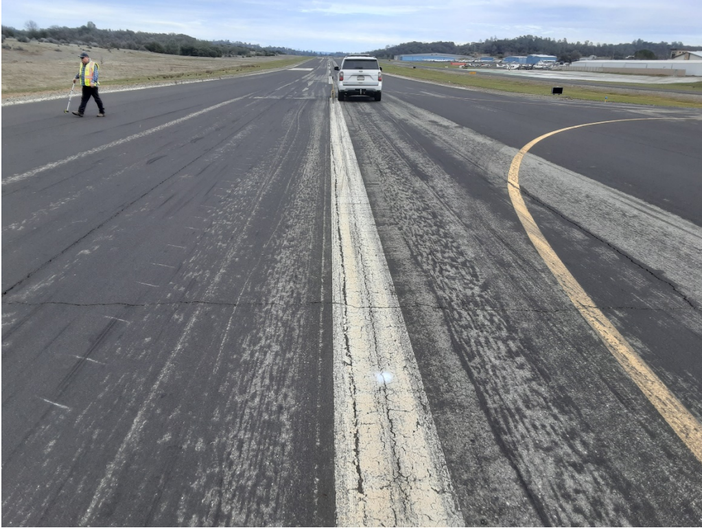
R1 B. LT cracking (Sample Unit No. 11).
