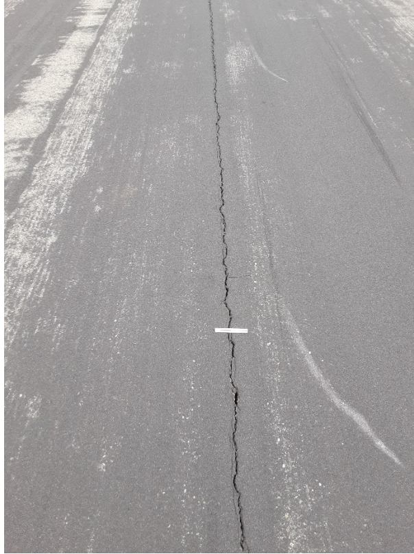
R1 B. LT cracking (Sample Unit No. 16).
