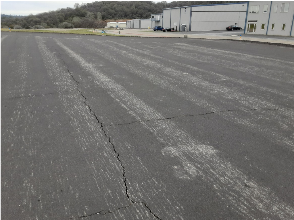
A6 A. LT cracking (Sample Unit No. 01).
