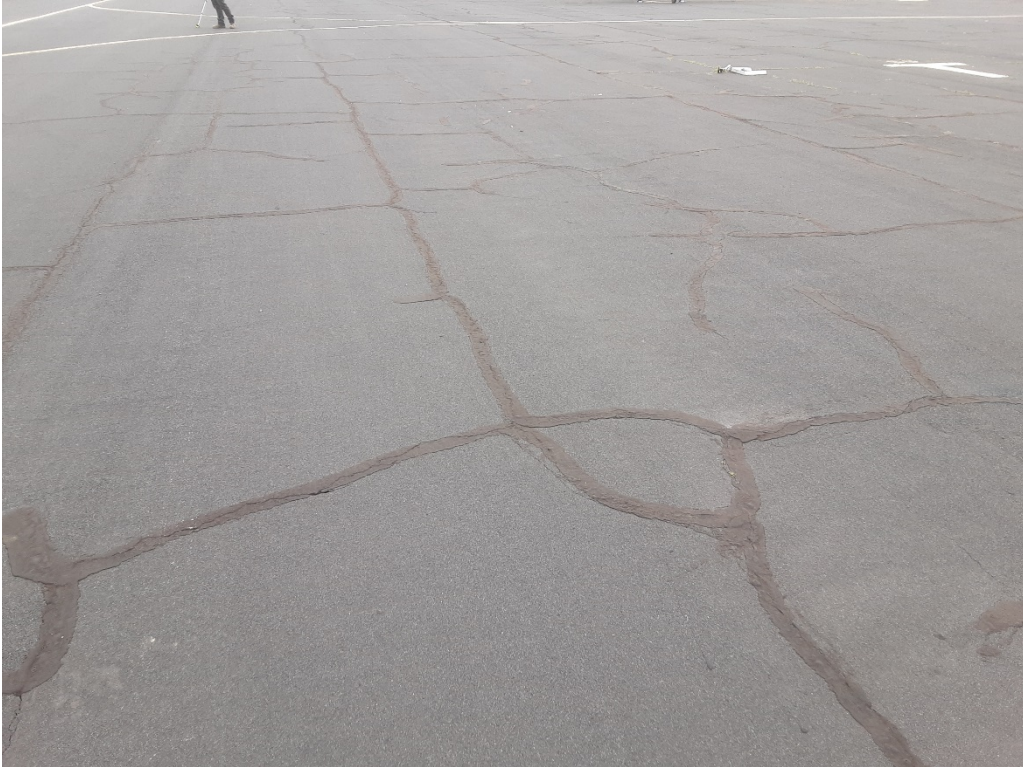
TD1 A. LT cracking (Sample Unit No. 06).
