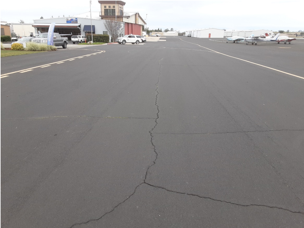
A2 A. Overview. LT cracking (Sample Unit No. 11).
