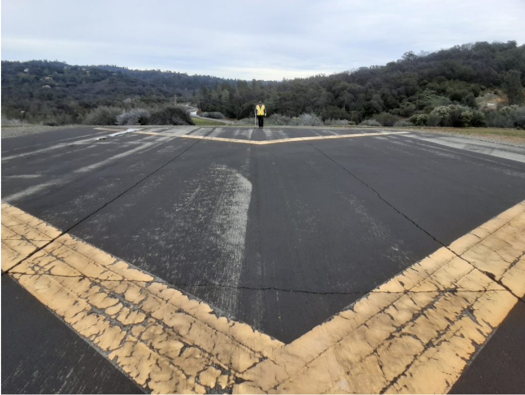
R1 C. LT cracking (Sample Unit No. 03).
