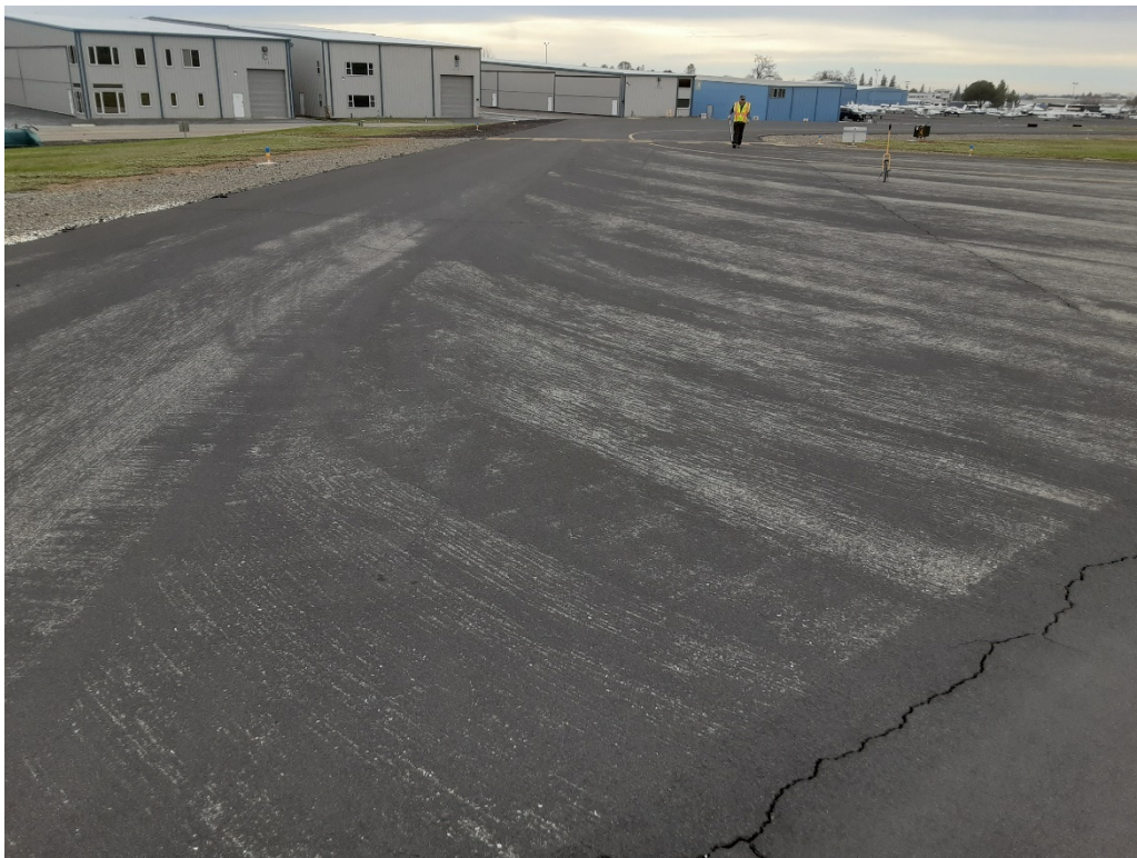
T7 A. LT cracking (Sample Unit No. 01).
