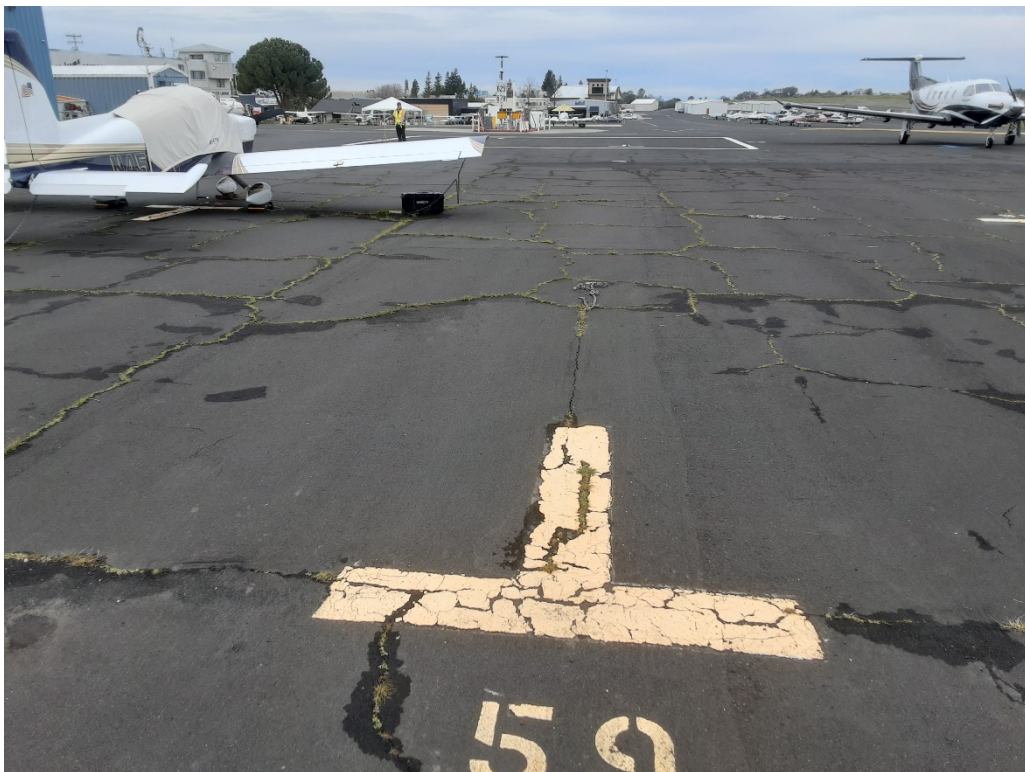
TD1 A. Block and LT cracking (Sample Unit No. 44).
