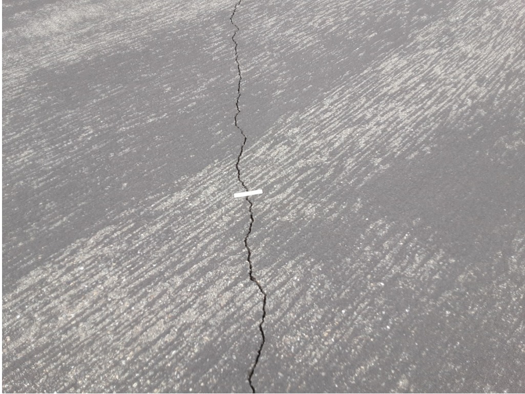
T7 A. LT cracking (Sample Unit No. 01).
