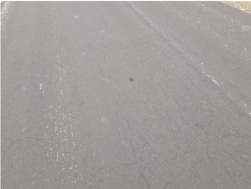
T1 A. Alligator cracking (Sample Unit No. 20).
