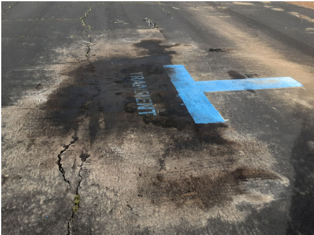
A3 A. Oil Spillage and LT cracking (Sample Unit No. 02).
