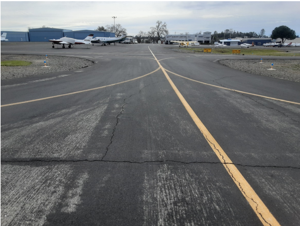
T8 B. LT cracking (Sample Unit No. 01).
