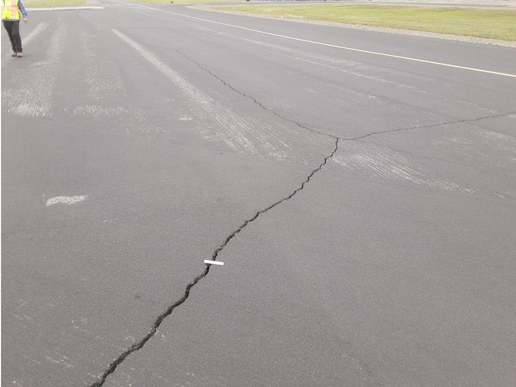
A6 A. LT cracking (Sample Unit No. 01).
