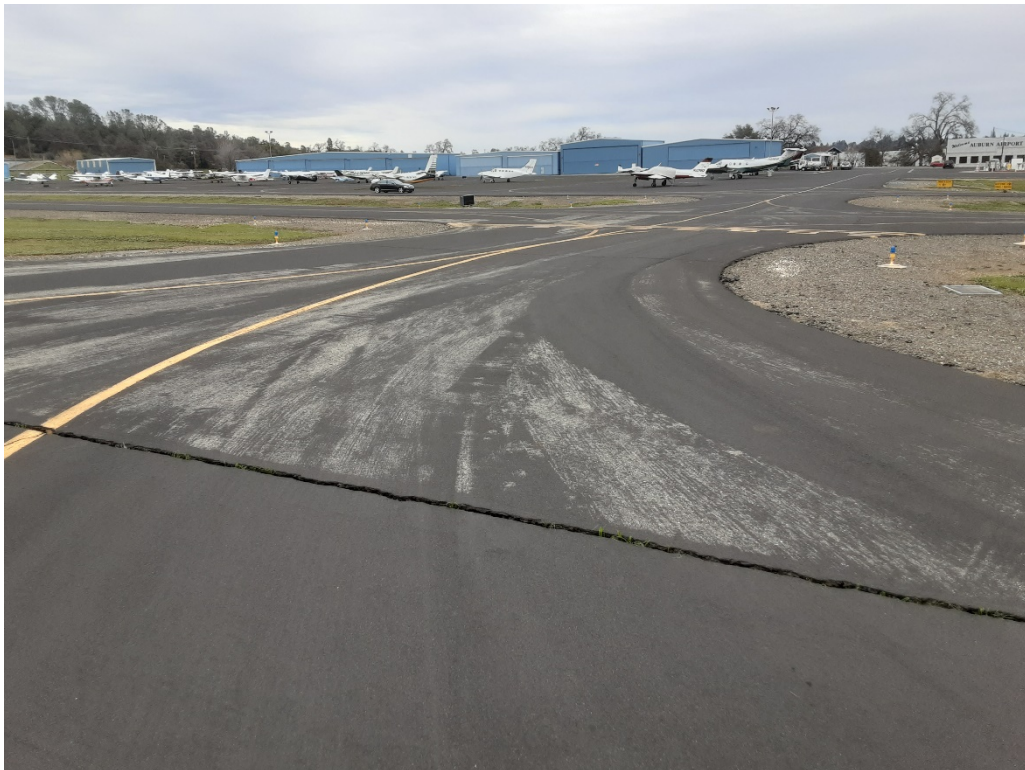
T8 A. LT cracking (Sample Unit No. 01).
