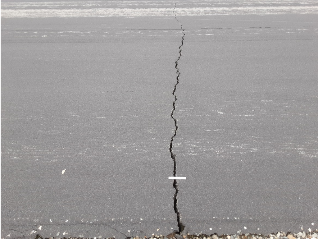
R1 B. LT cracking (Sample Unit No. 25).
