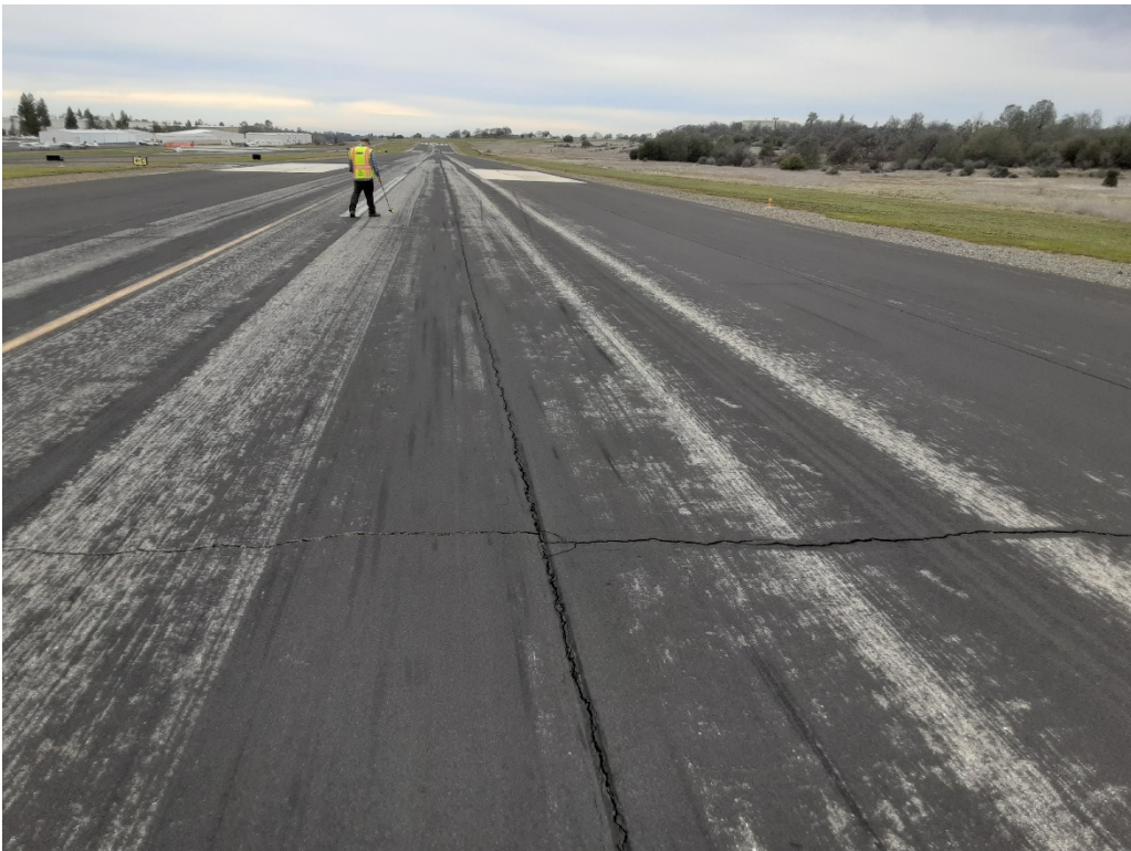
R1 B. LT cracking (Sample Unit No. 38).
