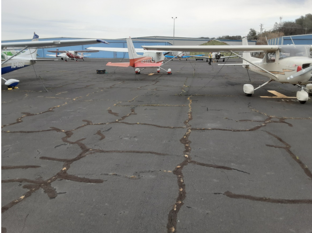
TD1 A. Block and LT cracking (Sample Unit No. 41).
