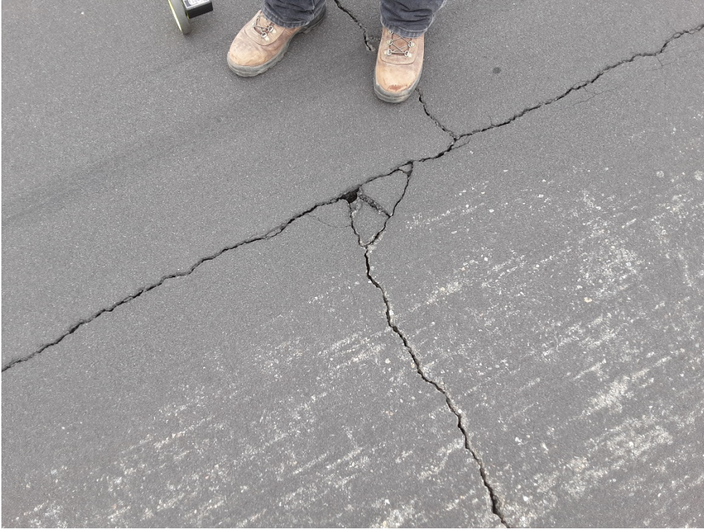
R1 B. LT cracking with the potential for pothole development and FOD (Sample Unit No. 29).
