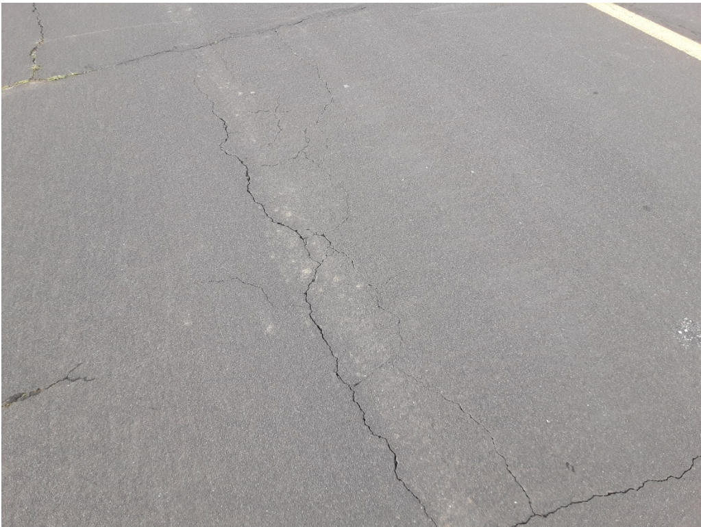
T5 A. Alligator and LT cracking (Sample Unit No. 02).
