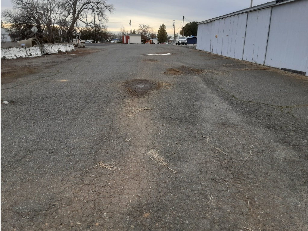
A9 A. Alligator cracking (Sample Unit No. 08).
