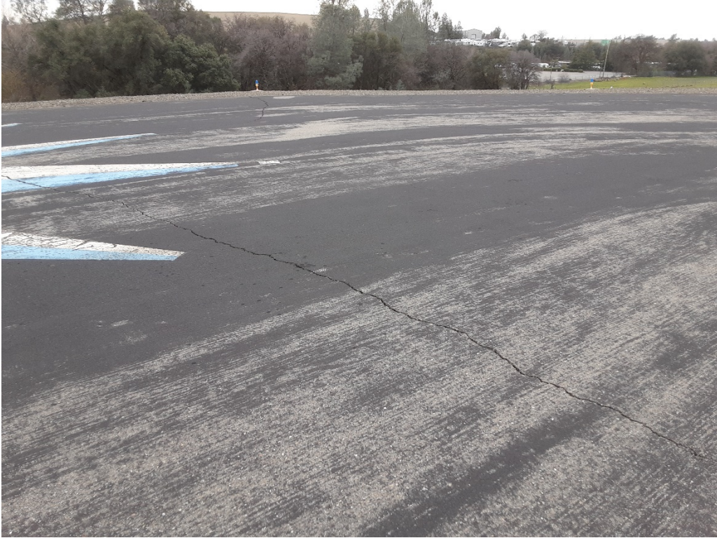
A5 A. LT cracking (Sample Unit No. 01).
