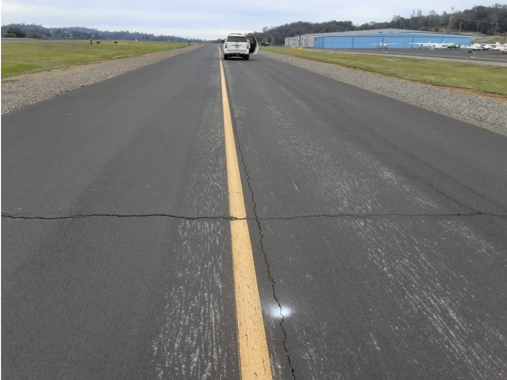
T1 A. LT cracking (Sample Unit No. 24).
