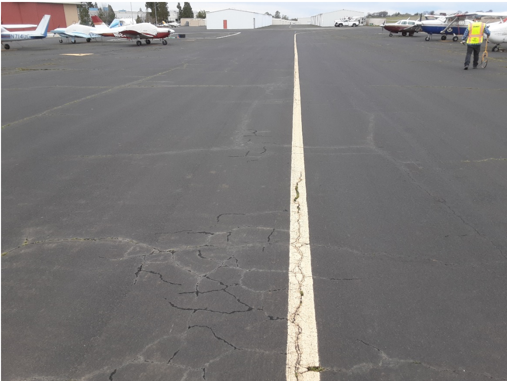
TD2 A. Alligator and LT cracking (Sample Unit No. 08).
