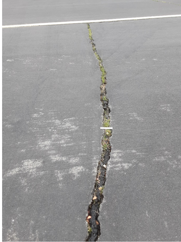
T6 B. LT cracking (Sample Unit No. 01).
