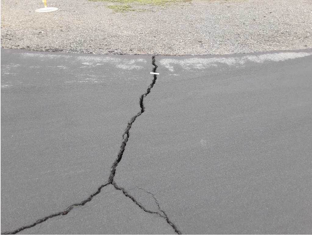
T1 A. LT cracking (Sample Unit No. 30).
