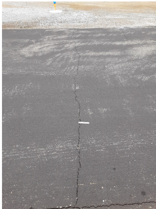
T2 B. LT cracking (Sample Unit No. 01).
