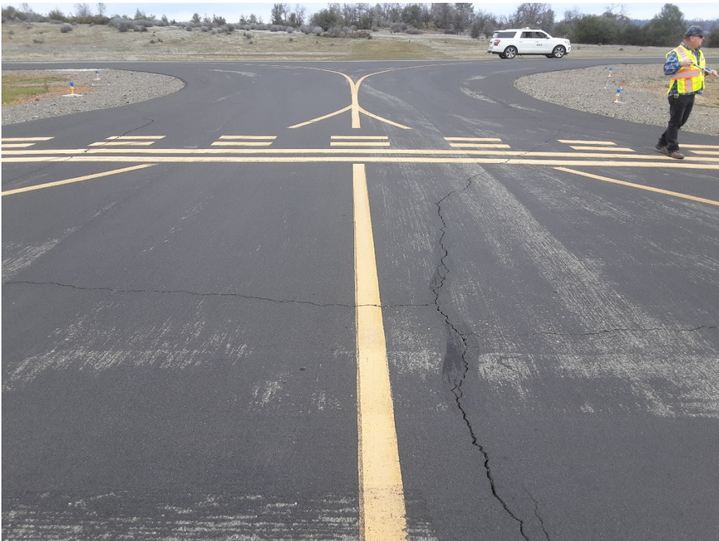
T2 A. LT cracking (Sample Unit No. 01).
