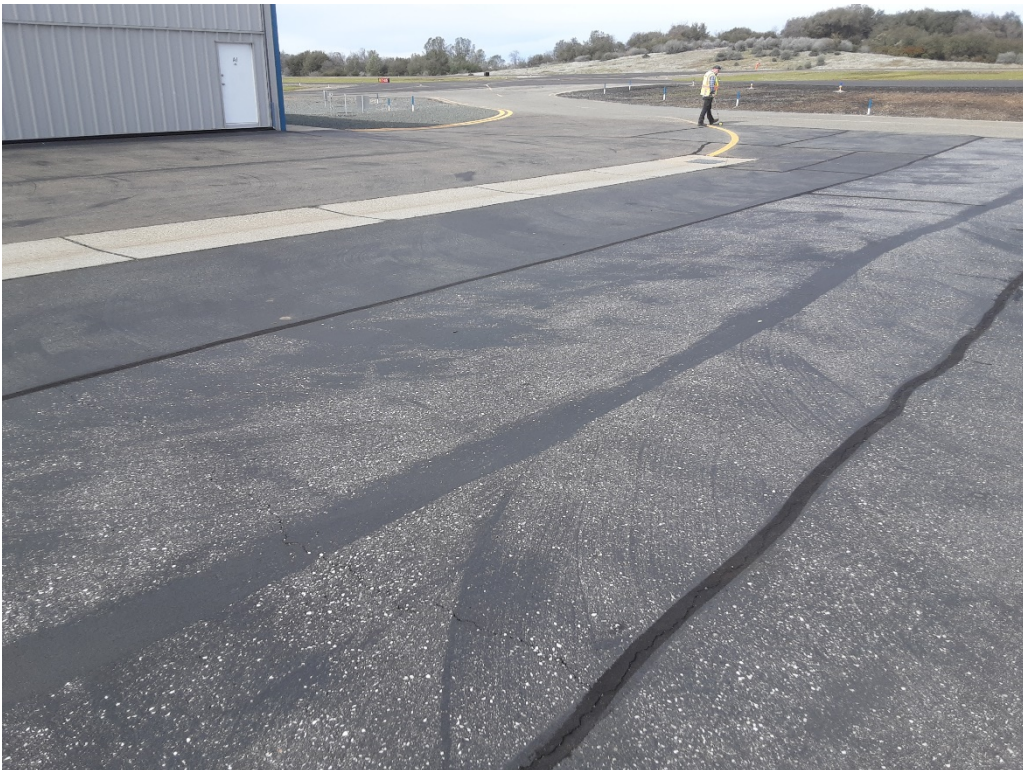
A8 A. LT cracking filled and bleeding (Sample Unite No. 06).
