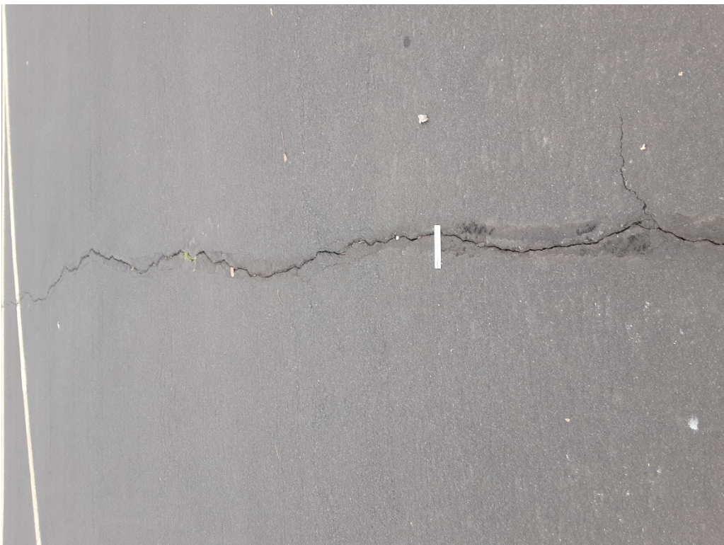
A2 A. LT cracking (Sample Unit No. 11).
