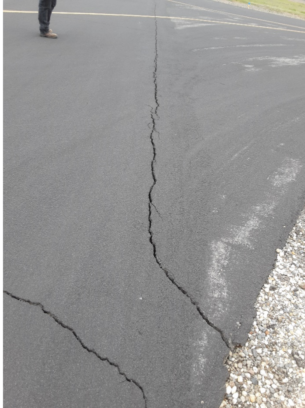
R1 B. LT cracking (Sample Unit No. 20).
