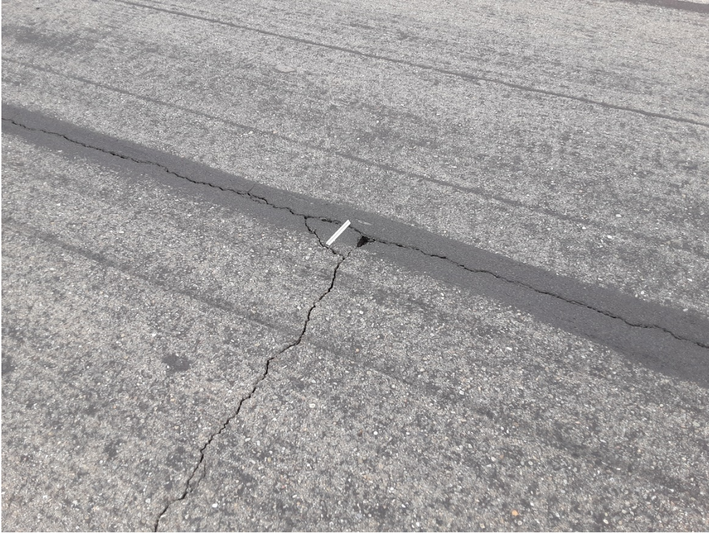
R1 B. LT cracking with the potential for pothole development and FOD (Sample Unit No. 34).
