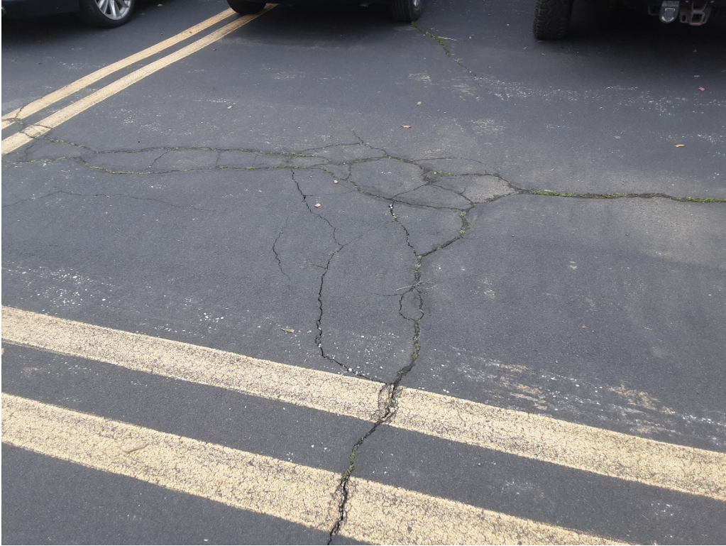
A1 A. Alligator cracking (Sample Unit No. 01)
