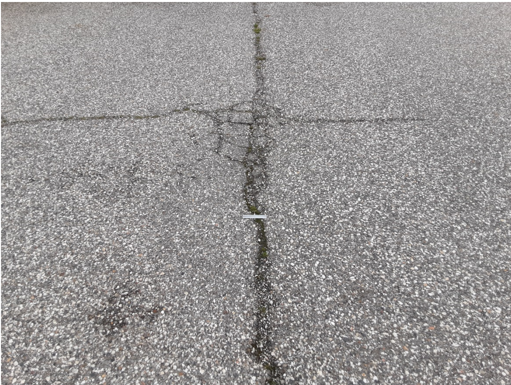
A7 A. LT cracking (Sample Unit No. 02)
