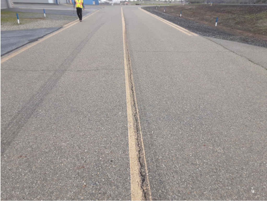
A8 A. LT cracking (Sample Unite No. 02).
