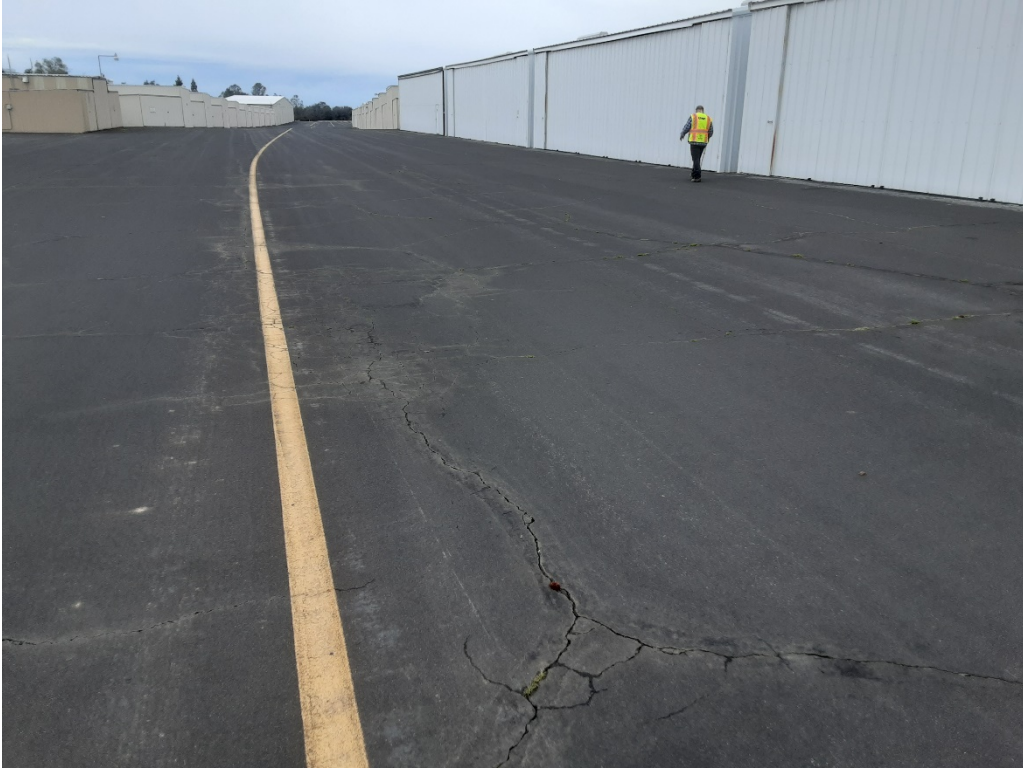
TD3 A. Alligator and LT cracking (Sample Unit No. 07).
