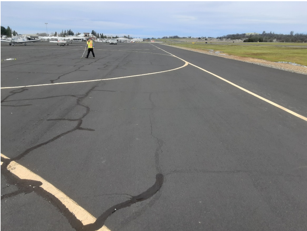
TD1 A. LT cracking (Sample Unit No. 06).
