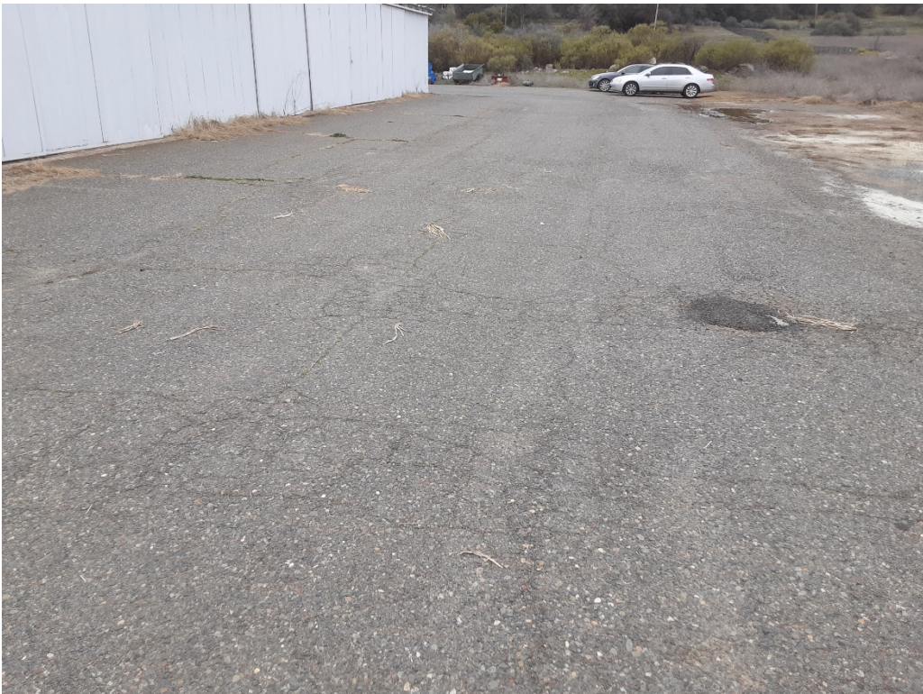
A9 A. Alligator cracking (Sample Unit No. 08).
