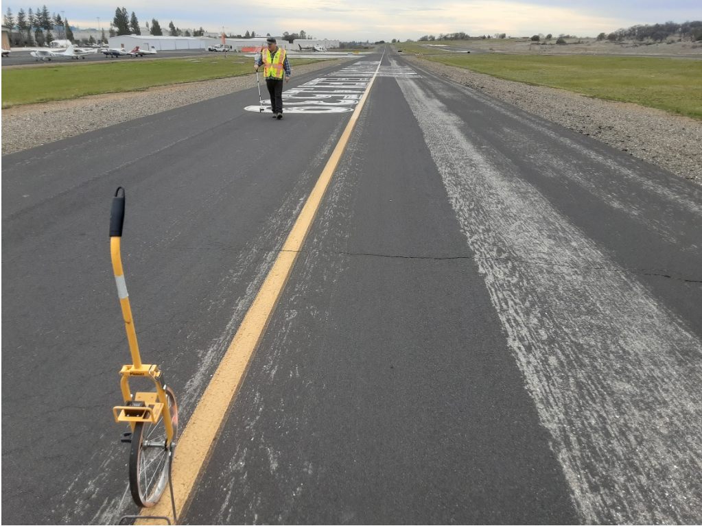
T1 A. LT cracking (Sample Unit No. 20).
