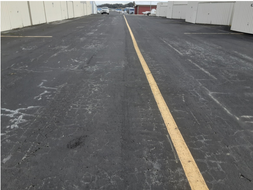
TD4 A. Alligator and LT cracking (Sample Unit No. 09).
