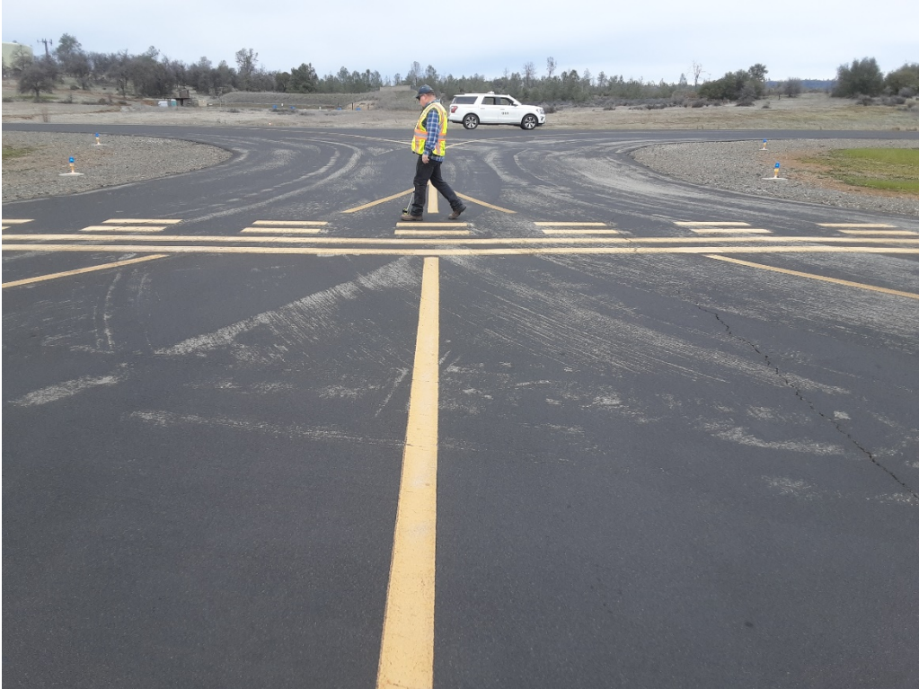
T6 A. LT cracking (Sample Unit No. 01).
