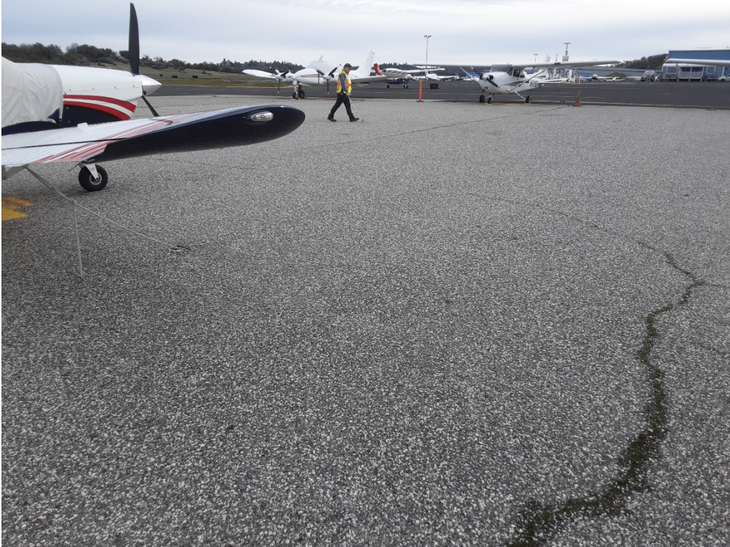
A7 A. LT cracking (Sample Unit No. 02)
