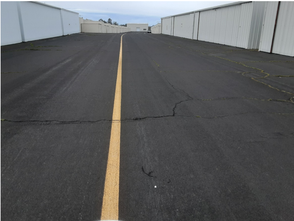
TD3 A. LT cracking (Sample Unit No. 12).
