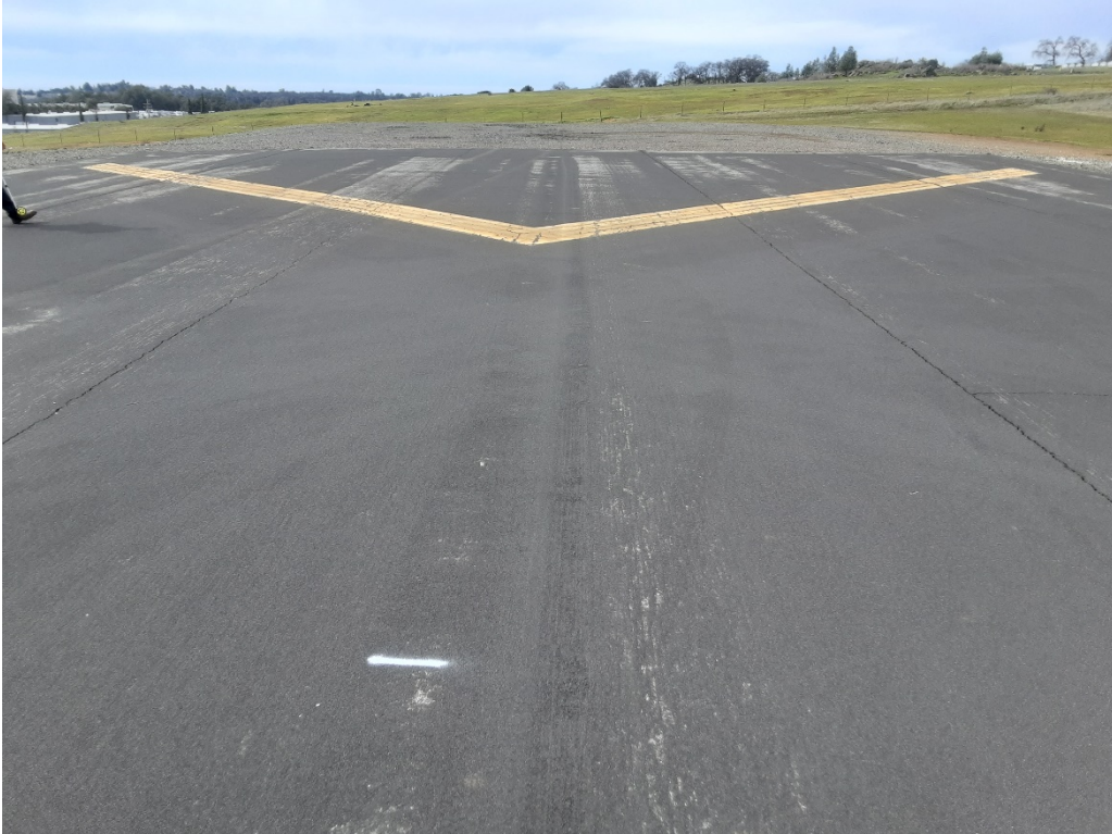
R1 A. LT cracking (Sample Unit No. 01).
