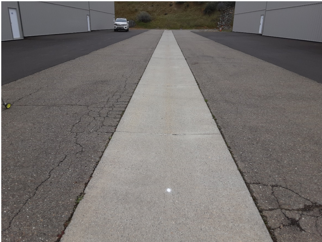
A8 A. Alligator cracking and LT cracking (Sample Unite No. 22).
