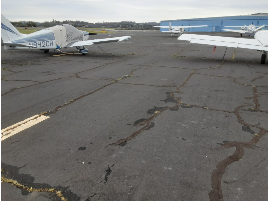
TD1 A. Block and LT cracking (Sample Unit No. 19).
