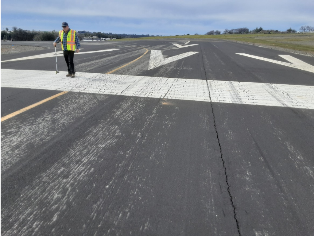
R1 B. LT cracking (Sample Unit No. 03).
