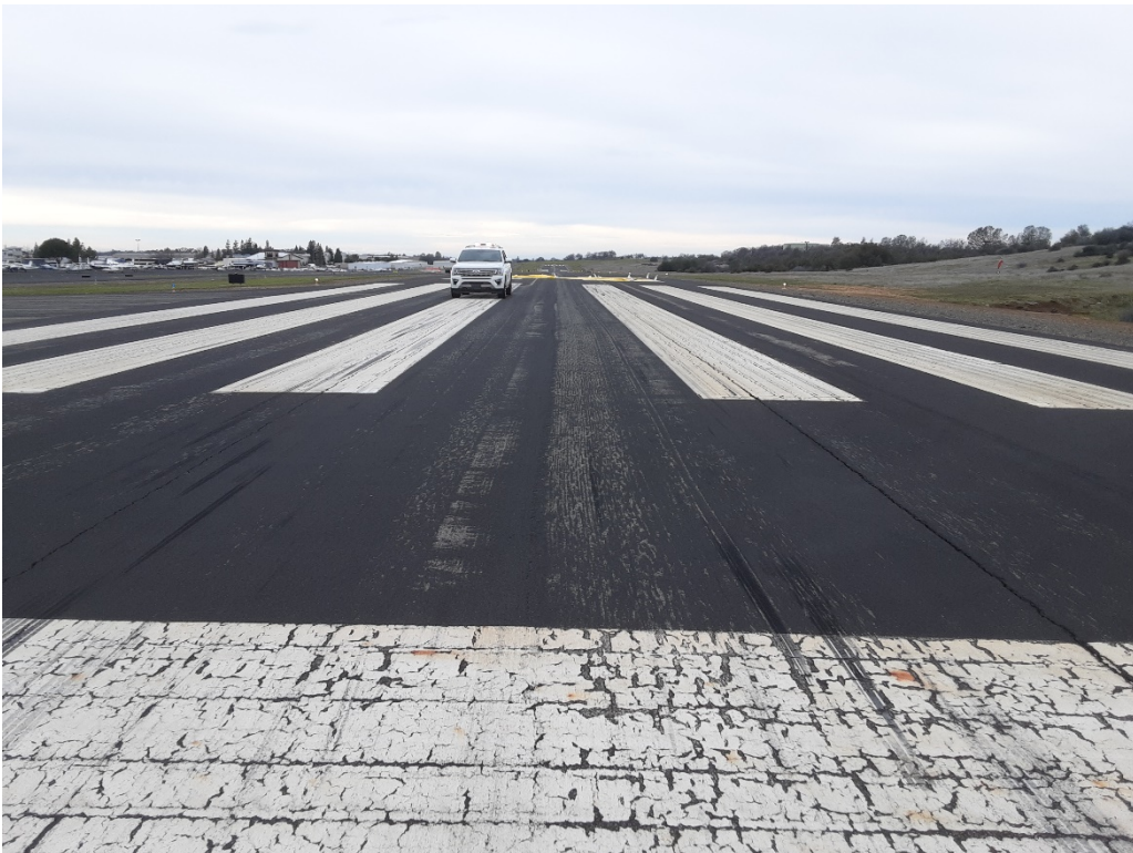
R1 B. LT cracking (Sample Unit No. 47).
