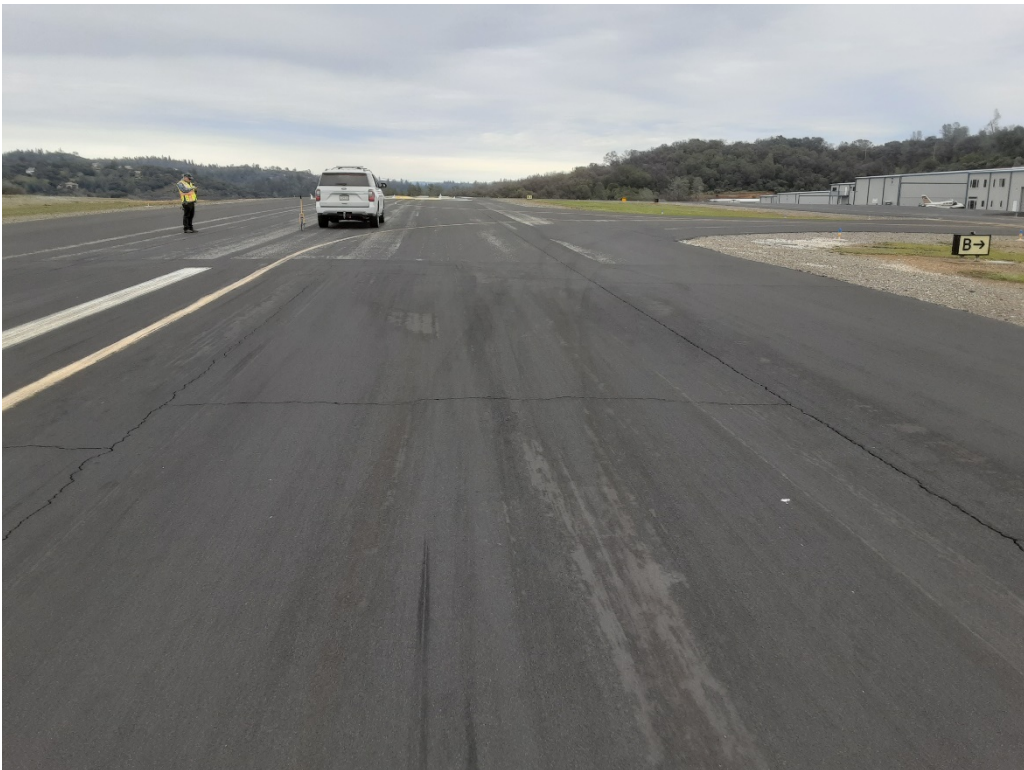
R1 B. LT cracking (Sample Unit No. 43).
