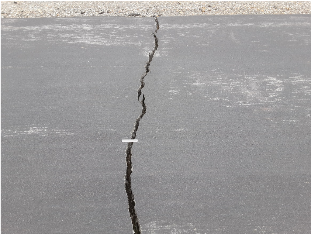
T1 A. LT cracking (Sample Unit No. 12).
