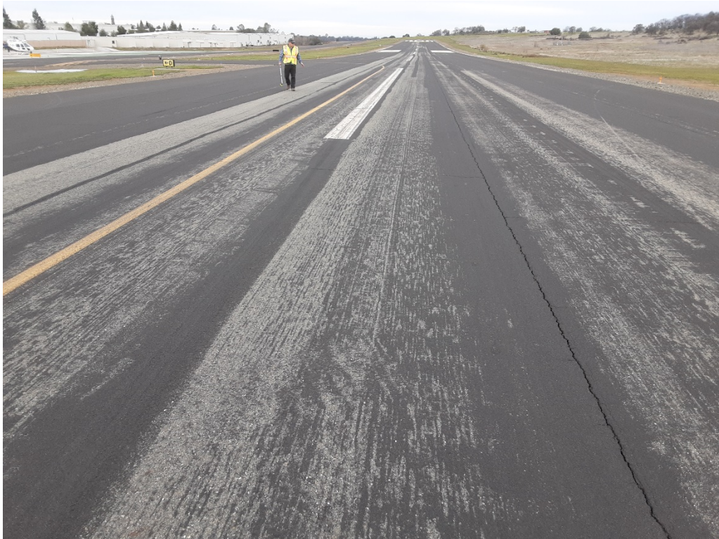
R1 B. LT cracking (Sample Unit No. 25).
