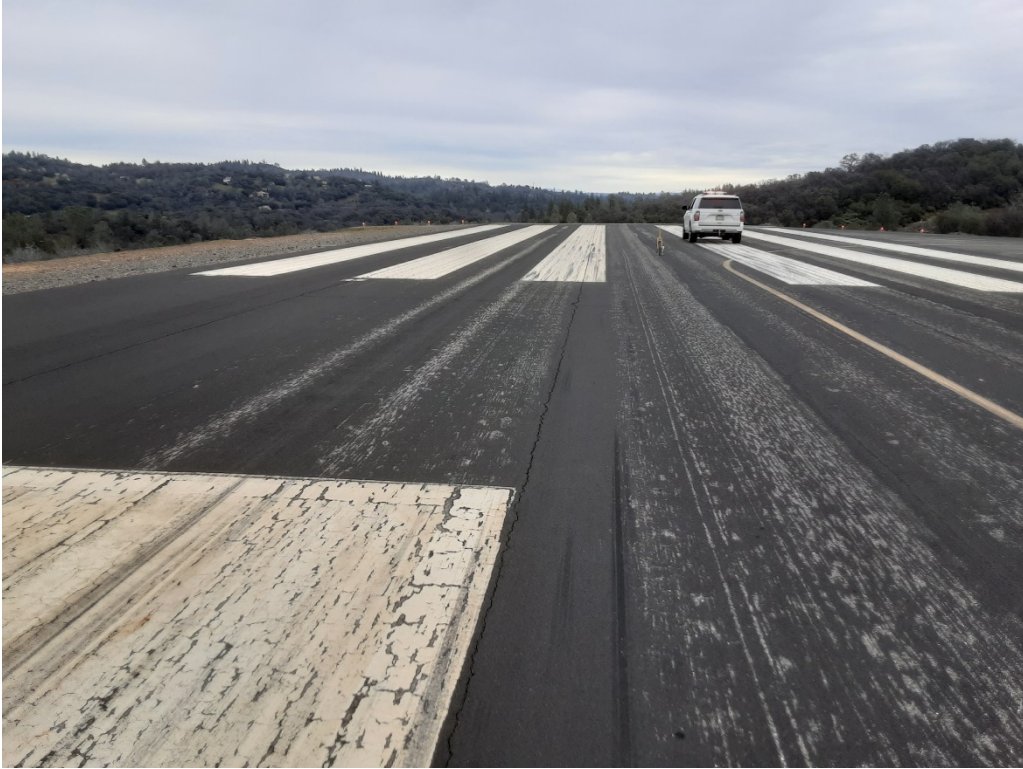
R1 B. LT cracking (Sample Unit No. 47).
