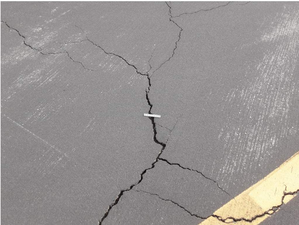
T4 B. LT cracking (Sample Unit No. 01).
